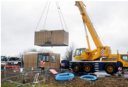
Repeat lifting operations
