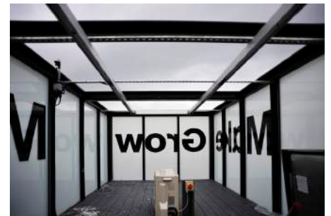
Fit-out and install lightbox glazing + signage
