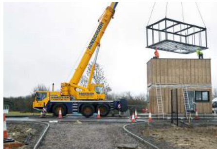
Crane lift of light-box module
