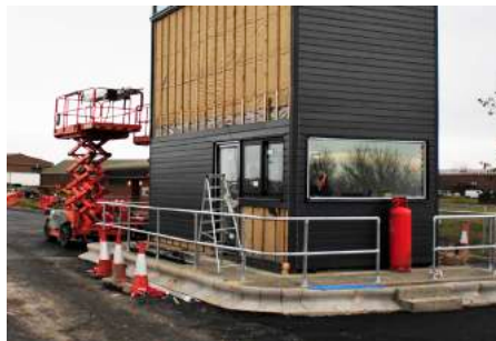
Clad in timber weatherboarding
