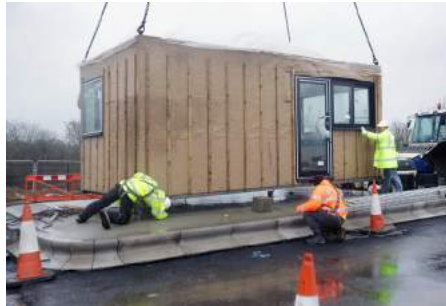
Locate onto capped-off services
