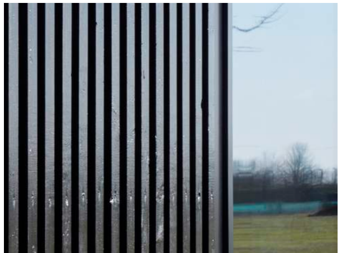
Black painted profile timber cladding at Alconbury Weald Club
