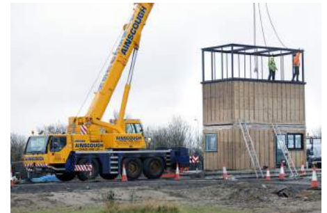
Fix light-box module to solid module
