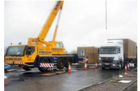
Second + third modules arrive by lorry
