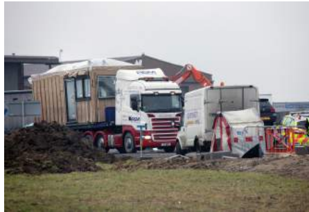
Prefabricated modules delivered by lorry
